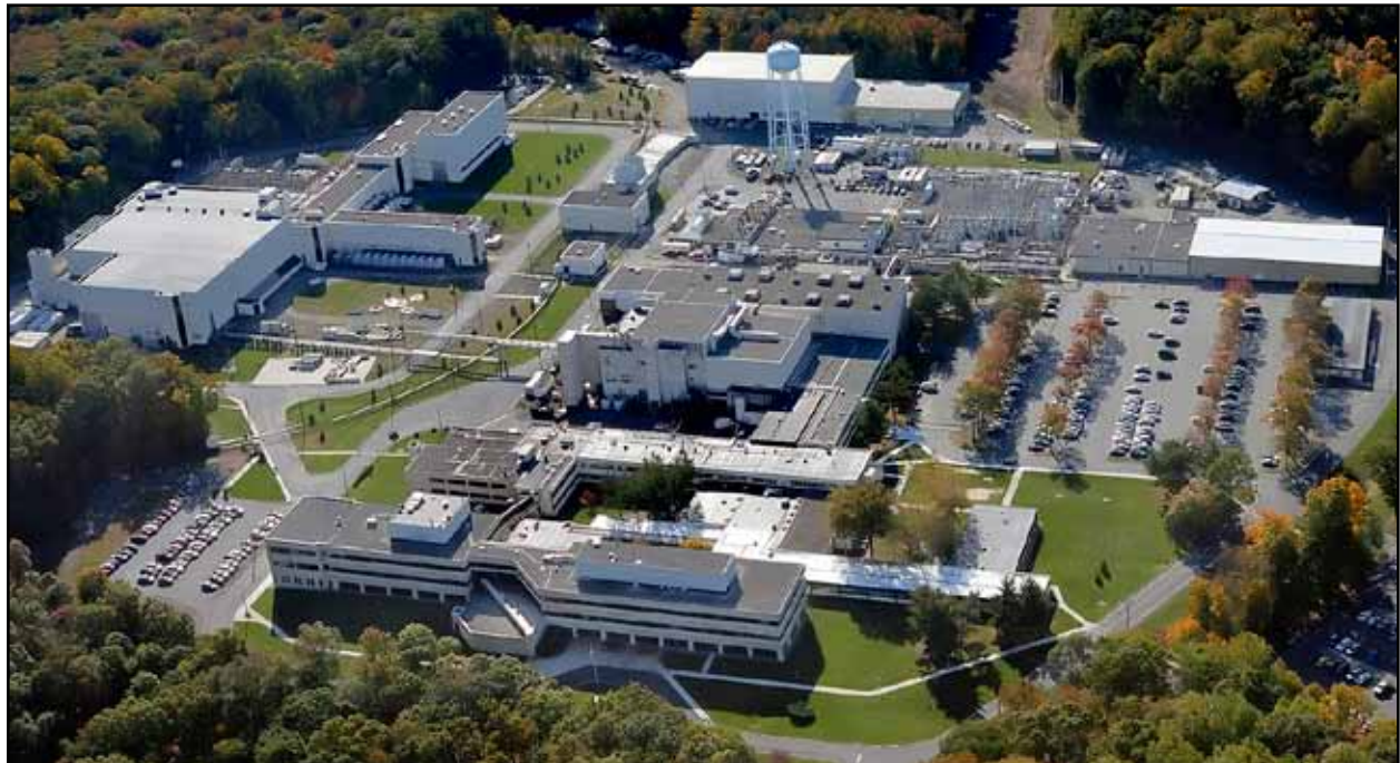
Aerial view of the U.S. Department of Energy's Princeton Plasma Physics Laboratory.
